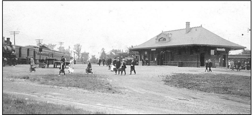
Freeville Railroad Station
